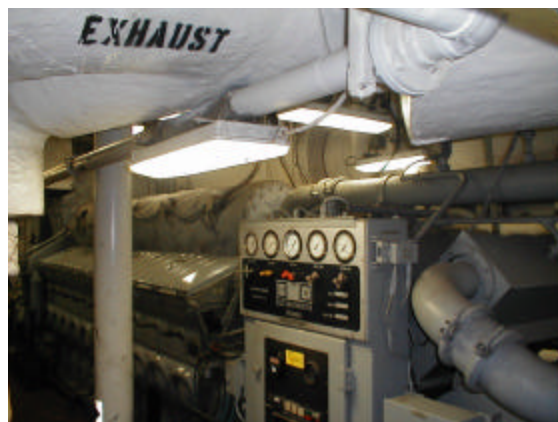
Engine Room After
