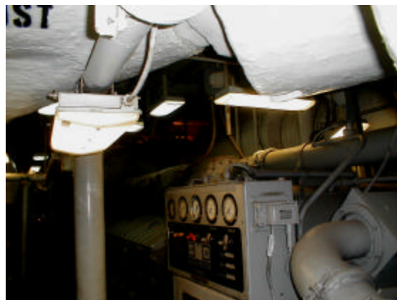
Engine Room Before
